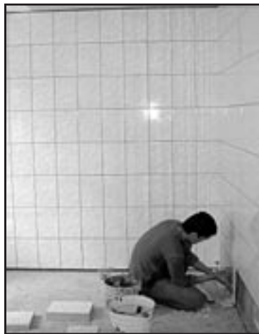
New tile being installed
